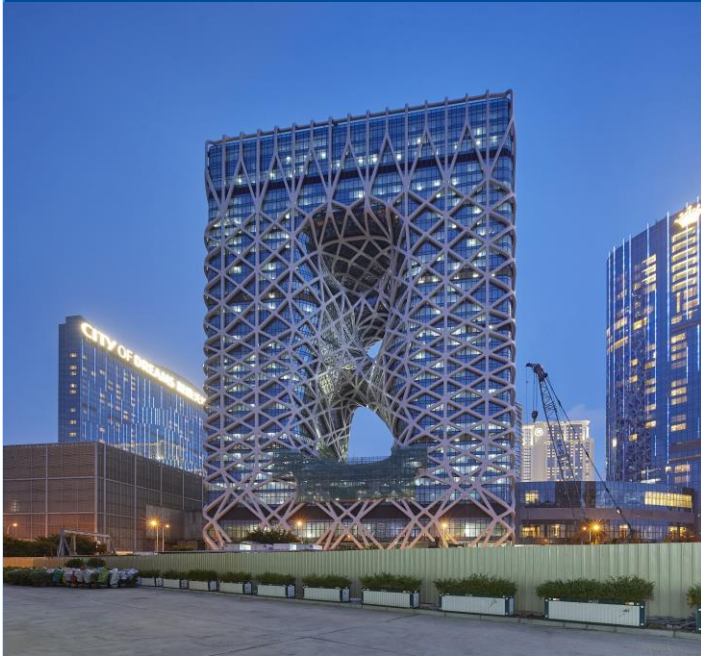
Image: Latest Construction Update
